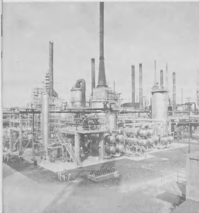
and new HDS-II unit on the "flats" is the Virgin Naphtha Hydrofiner. Unidad nobo di HDS-II ta Virgin Naphtha Hydrofiner (N2AR).
